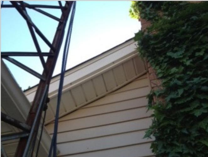
Soffit after rebuilding after Raccoon damage
